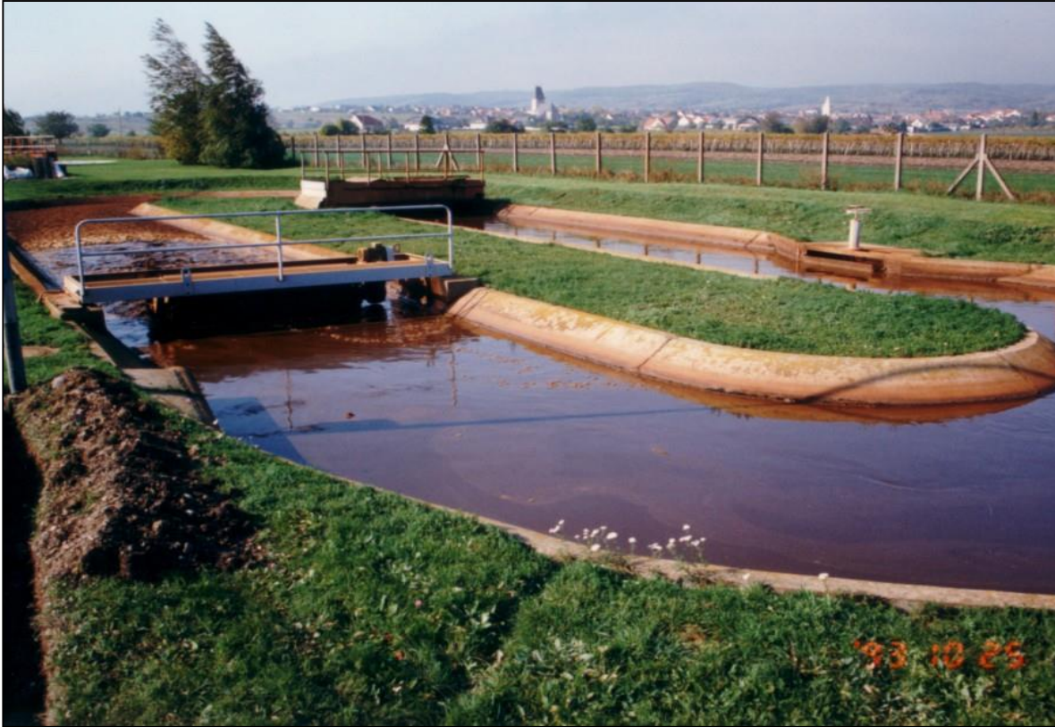
Aeration rotors \varnothing 700mm
